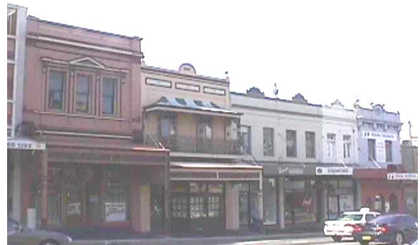
Photo: Commercial buildings along Parramatta Road.
