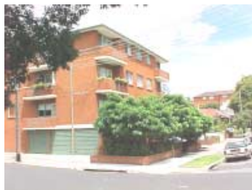
Photo: 3-storey walk-up flats in the area bounded by Regent, Flood, Marion and Edith Streets.
