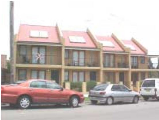
Photo: The two-storey townhouses along Darley Road, with good use of appropriate building materials, side gabled iron roofs, and low brick/iron fencing.
